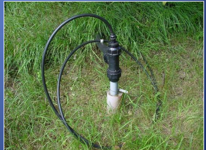
Obr. 9: Bioremediace: detail vrtu bioventingu
