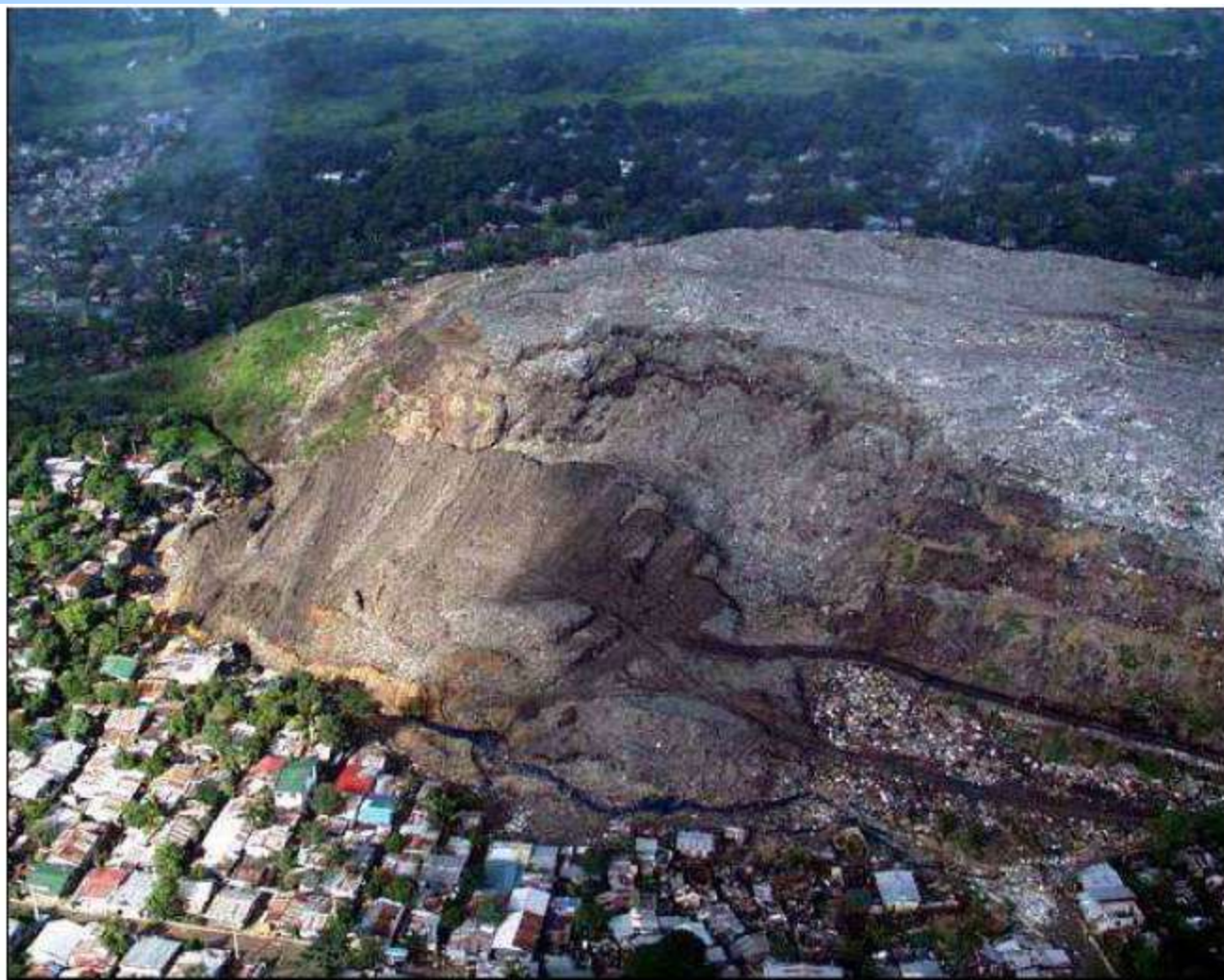
Figure 1-2 Aerial View of Payatas landfill (Philippines) failure (Source: Zekkos, 2005)
